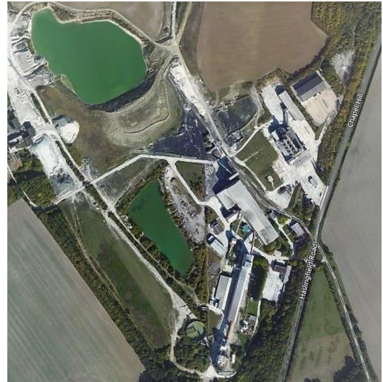
Barrington Cement Works, Cambridge
