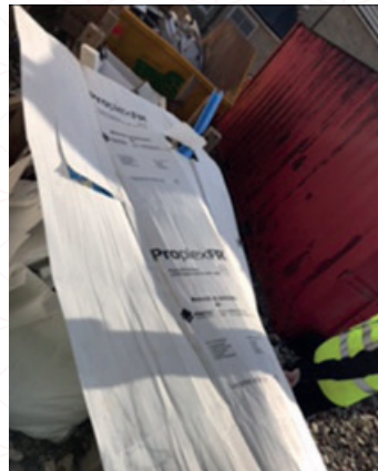
Temporary protection sheet disposed of in waste from plot 136 Yorkshire.
