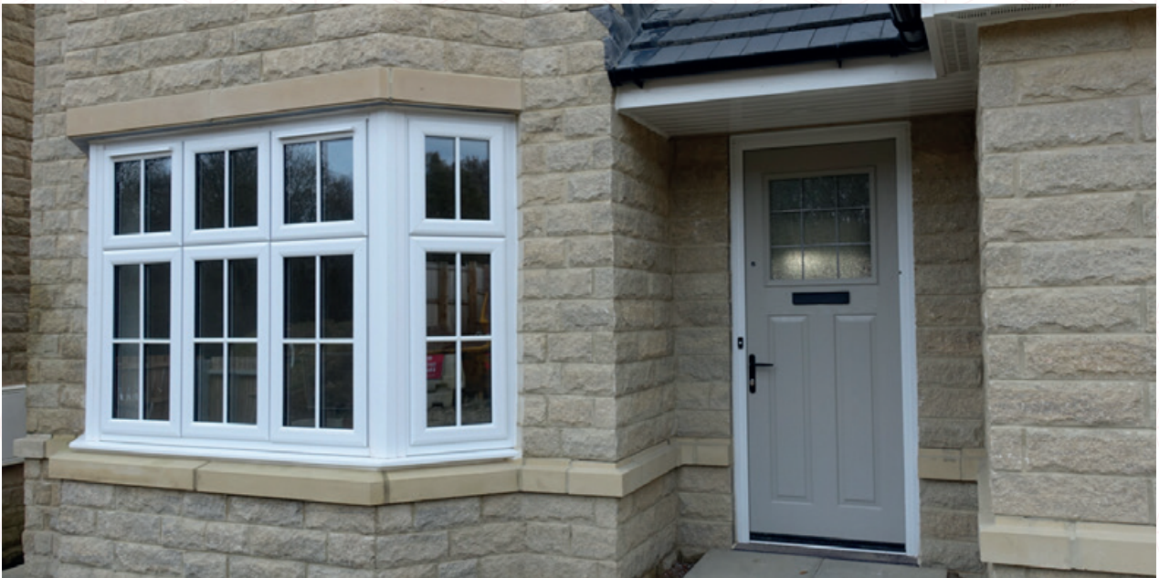
Bay windows of the Oxford Housetype
