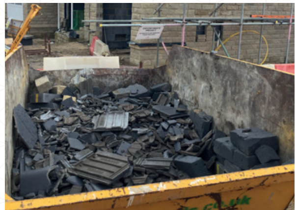
Damaged tiles/inert waste from plot 136, Yorkshire.
