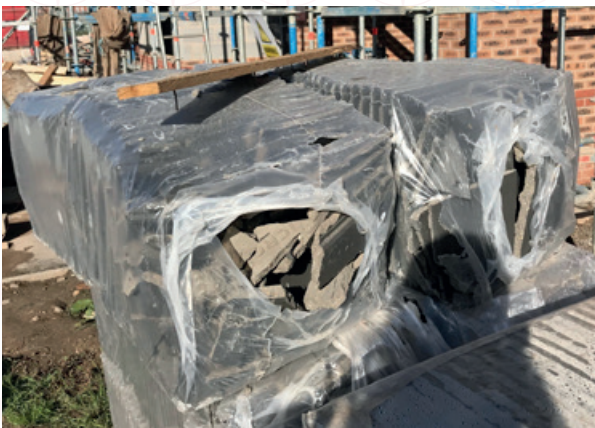
Damaged roof tile delivery to the Brook, Lancashire.
