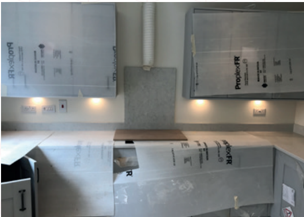
Temporary protection sheets used to protect kitchen in plot 121 Lancashire.
