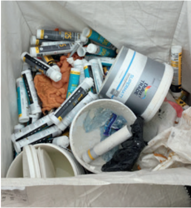
Hazardous material product packaging waste (3 paint tins, approx. 60 mastic tubes and expander foam containers). 1 bag, total weight = 25kg.
