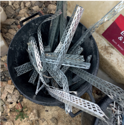
Plasterboard angle bead
