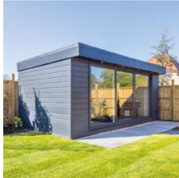
Garden Pod, Ash Holt at Newton Garden Village, Nottinghamshire
