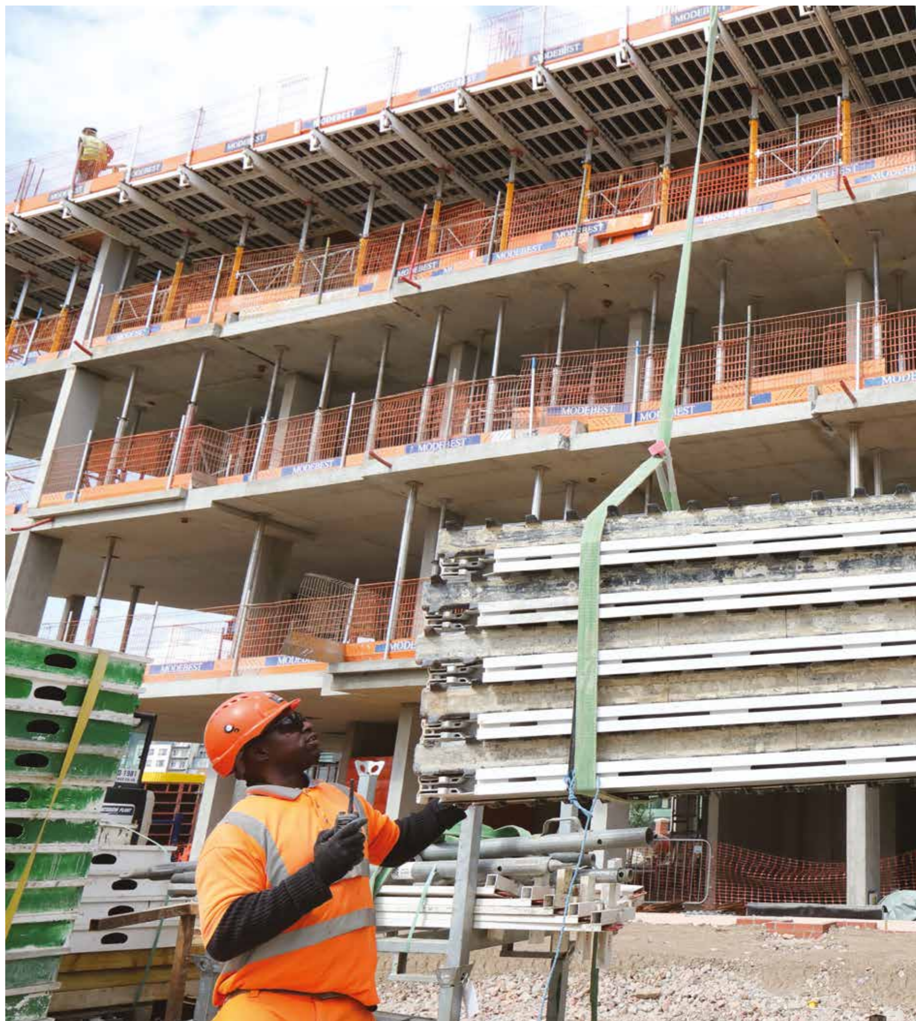
CONSTRUCTION IN PROGRESS AT COLINDALE GARDENS, LONDON
