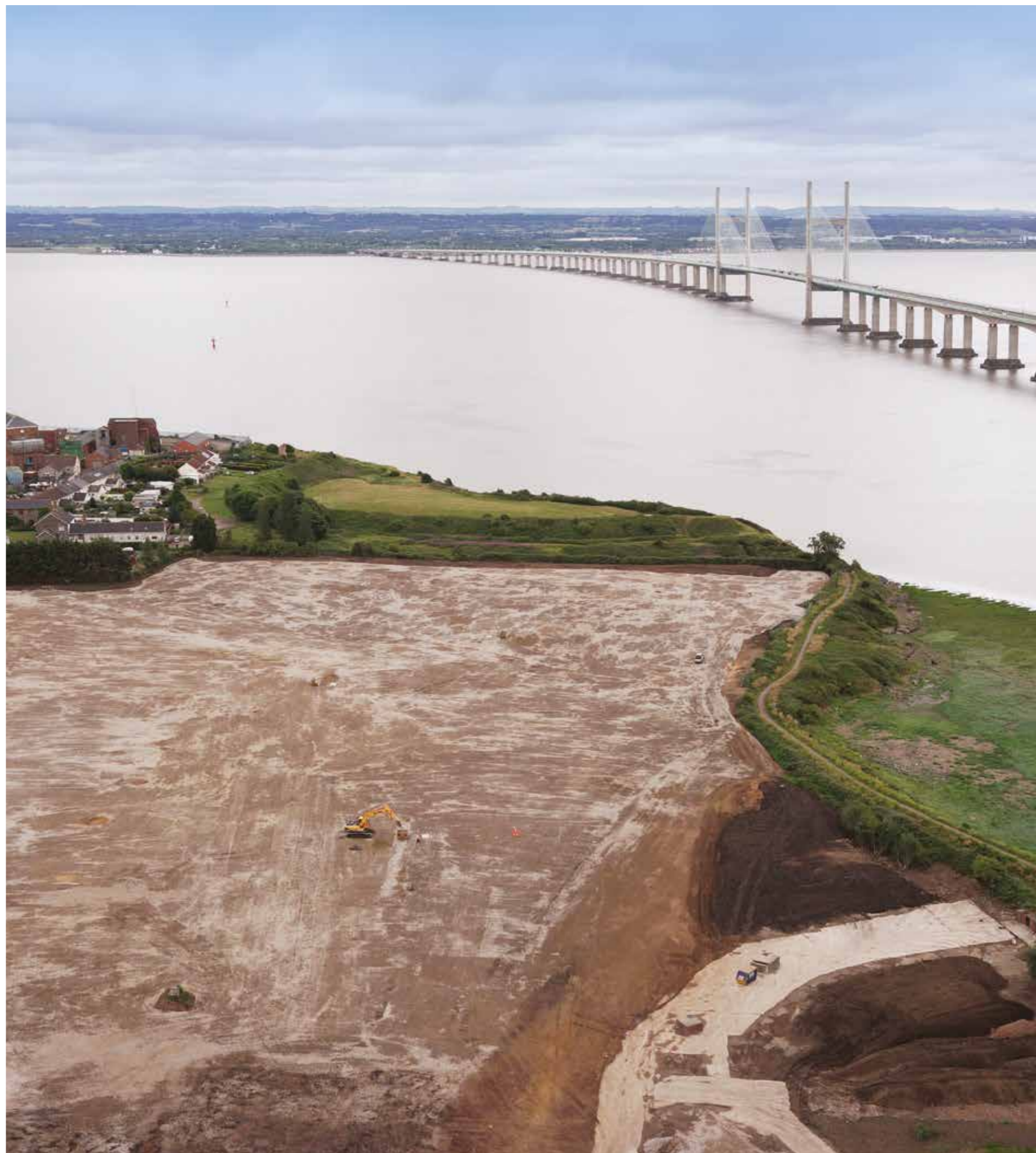
REGENERATING A BROWNFIELD SITE AT SUDBROOK, MONMOUTH
